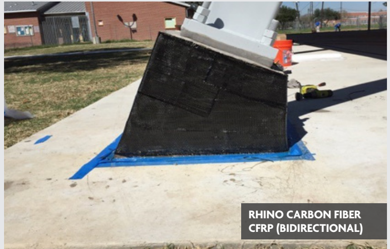
CRACKED THRUST BLOCK
