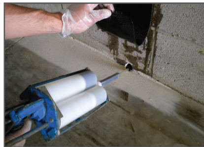
Apply epoxy to hole
