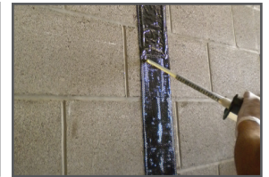
03: Apply carbon fiber strap & coat with epoxy
