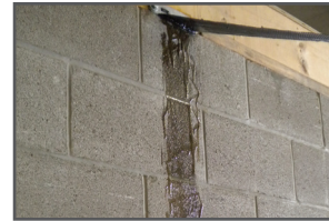
02: Spread epoxy on foundation wall
