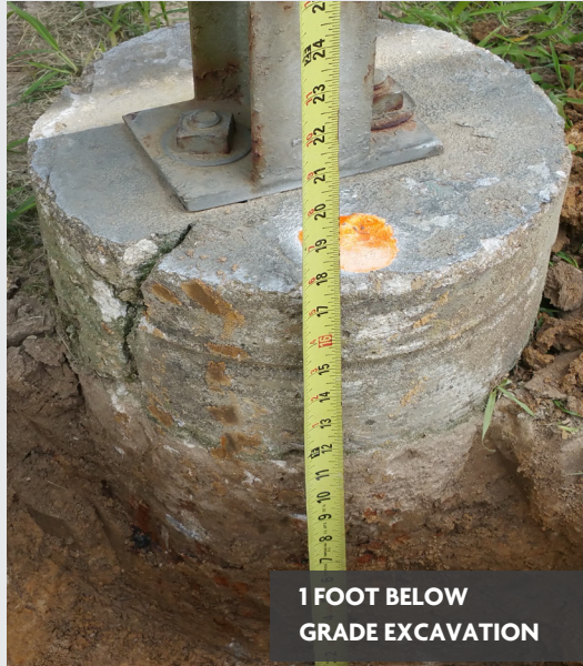
CRACKED CONCRETE SUPPORT
