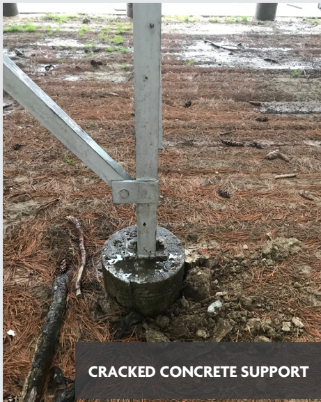
CRACKED CONCRETE SUPPORT
