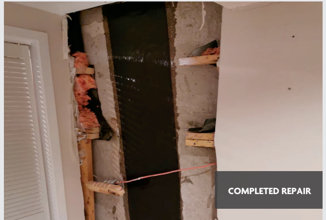
CFRP APPLICATION
