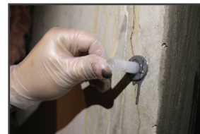
02: Press port firmly directly over crack
