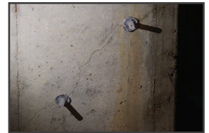
03: Cover over previously marked locations
