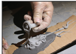
01: Roll port edge in High Strength Anchoring Epoxy Paste
