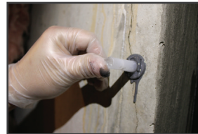
02: Press port firmly directly over crack
