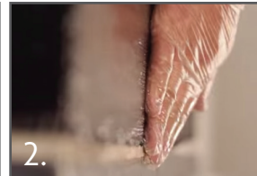
2. Work carbon fiber into epoxy. Add more epoxy if necessary
