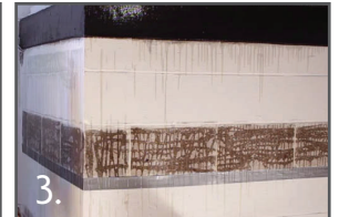
3. Repeat process to additional sections
