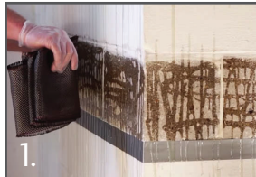
1. Mount carbon fiber to the wall
