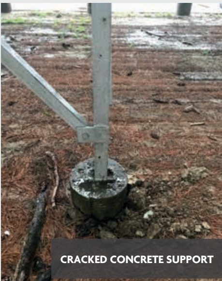
CRACKED CONCRETE SUPPORT
