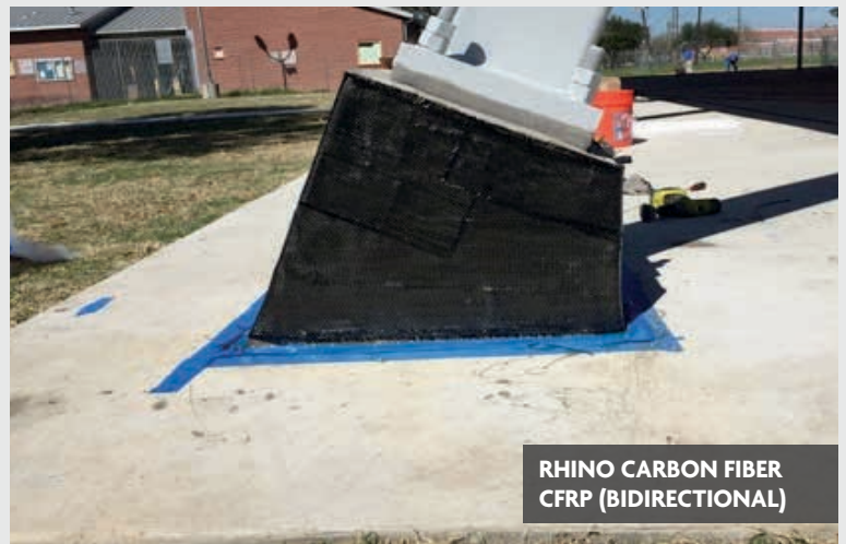
CRACKED THRUST BLOCK
