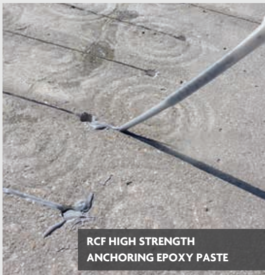
RHINO CARBON FIBER CONCRETE CRACK LOCK® STITCH
