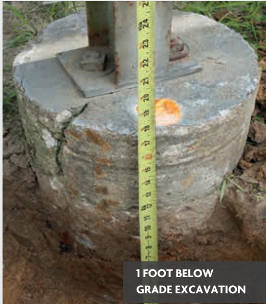
CRACKED CONCRETE SUPPORT
