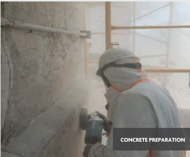
SCAFFOLDINGS FOR PREP/INSTALL
