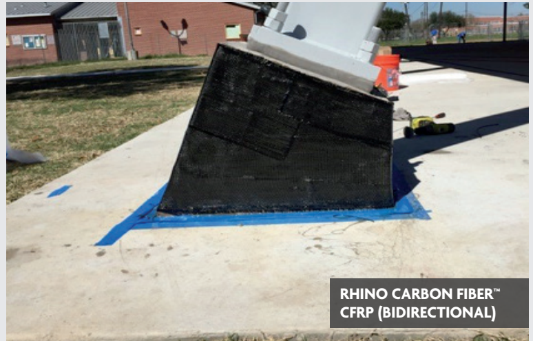
CRACKED THRUST BLOCK
